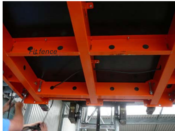
Lead the cables through the platform
